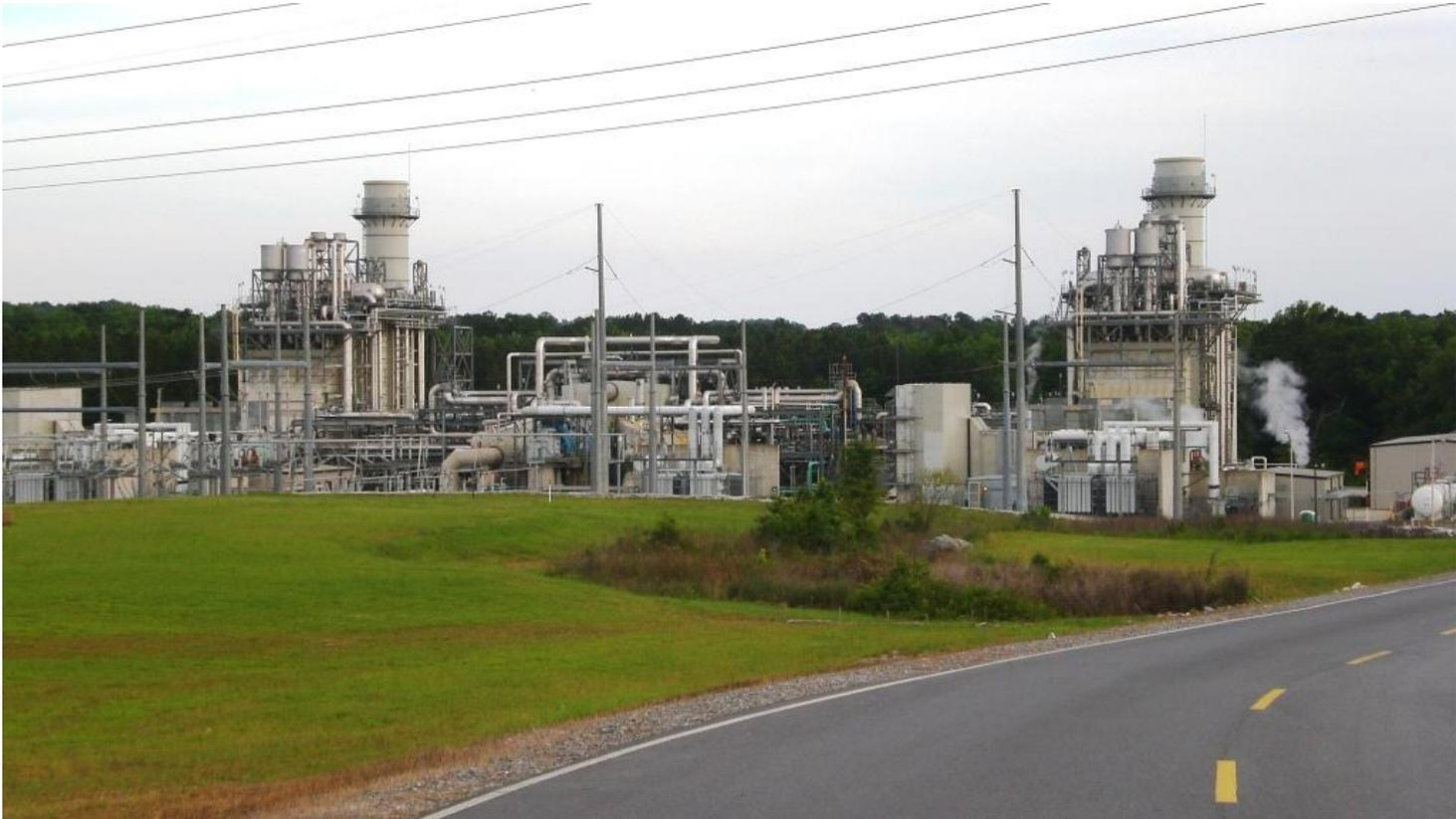
**Facility Type:** Combined Cycle Natural Gas Power Plant (670 megawatt)
