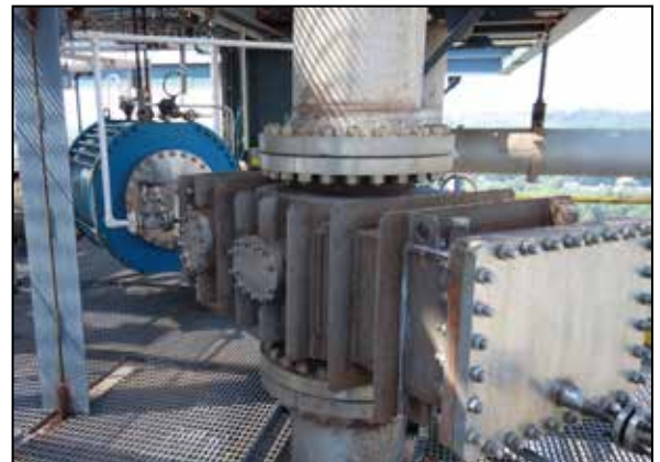
Double Disc Valve in FCC Service
