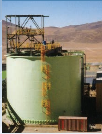
LHX-13C operating on a 59' diameter copper concentrate slurry surge tank.
